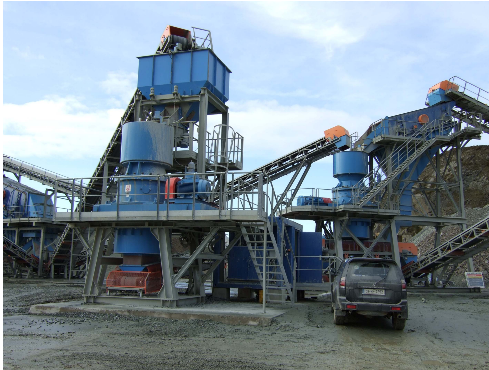
Fig 11 – Secondary crusher (200kW motor) in foreground. Primary unit is in the right background
