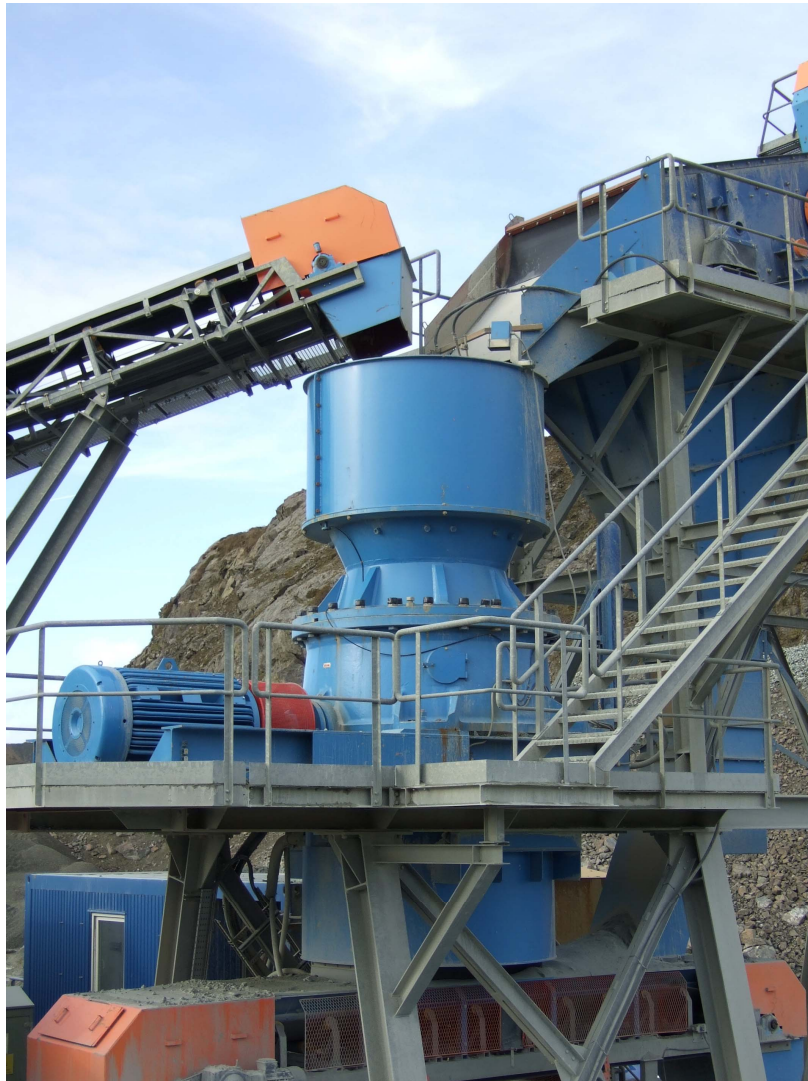
Fig 5 – Cone crusher with 315kW induction motor with active filter
