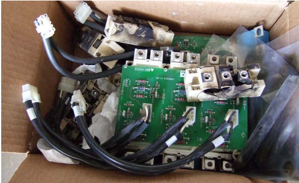
Fig 16 : Result of repetitive voltage spikes. Diode packs destroyed and DC bus capacitors destroyed in shaker VFDs.
