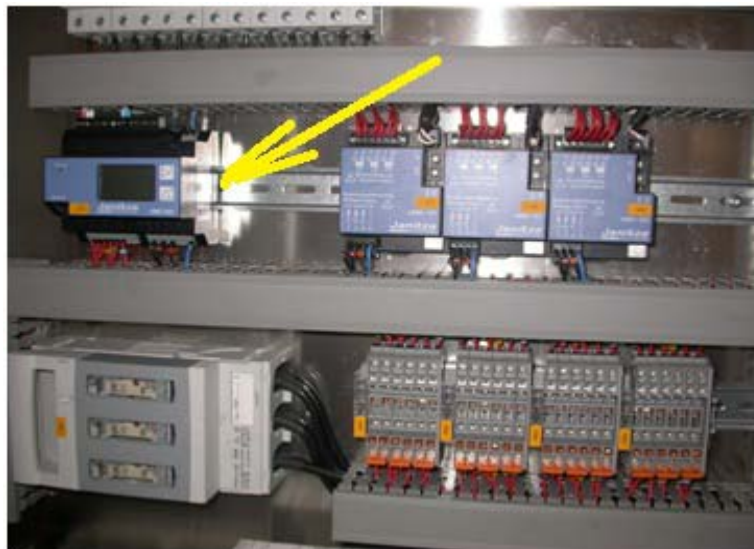
Fig 28 : Power quality monitor installed in switchboard
