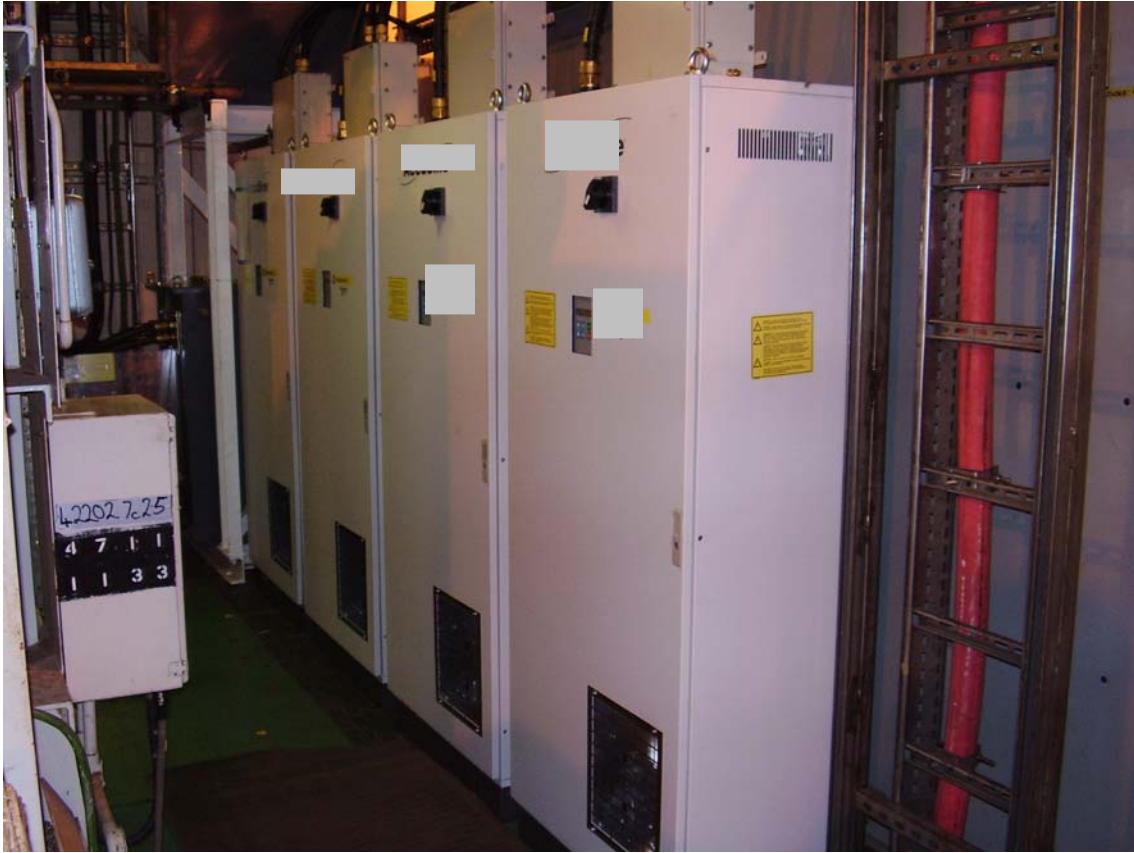
Fig 14 – 4 x 300A active harmonic filters on offshore oil platform
