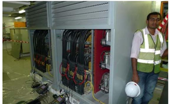
Fig 15 : 2 x 2300HP/1800kW D type wide spectrum filters on mud pumps during ABS compliance testing in the UAE
